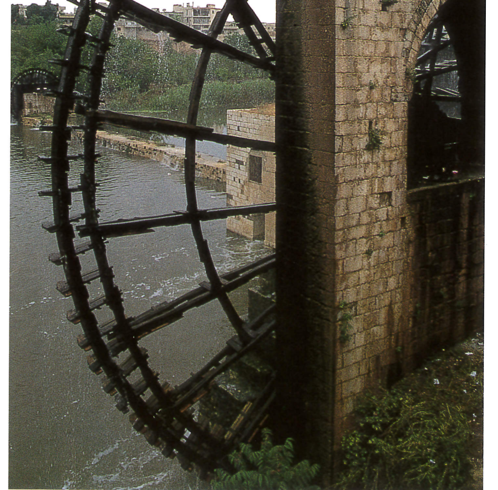
WATERWHEELS Bringing water into the city was sometimes a major task. In Hamah, Syria, two huge wooden waterwheels mounted on massive stone arches were built to raise water from the river to supply the town. Building wheels like this required great engineering skill.
